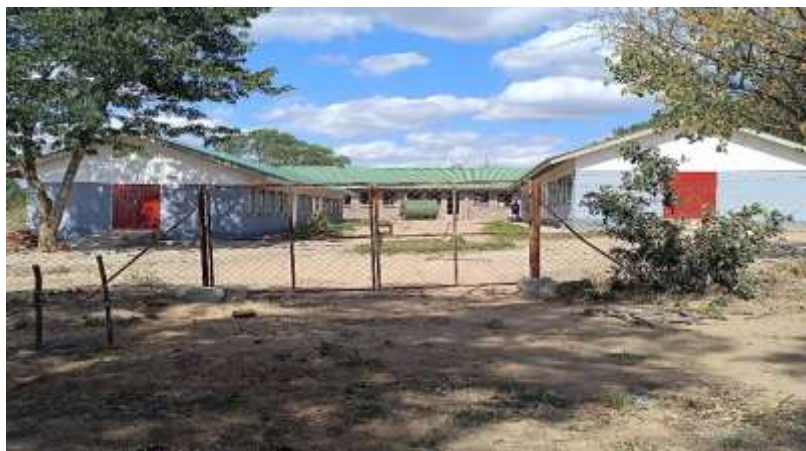
Figure 1 Shows the new mother's shelter under construction at the Hospital
